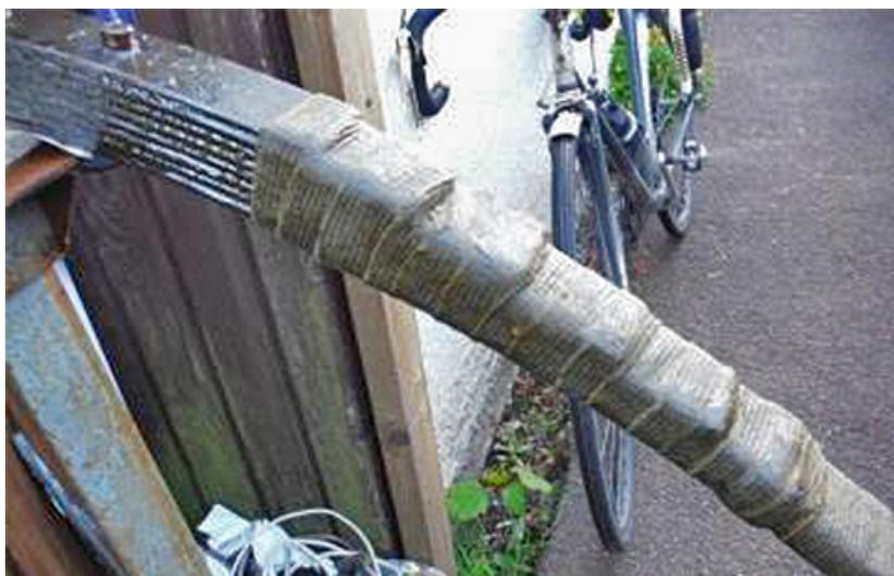
After greasing, reassembly and taping
